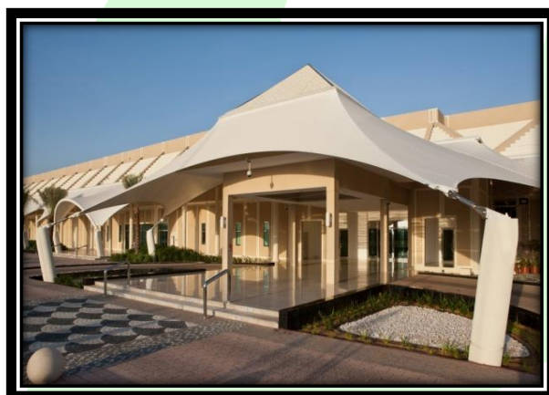
CCU SUPPLY & INSTALLTION WORKS AT ADNEC – ALAIN
