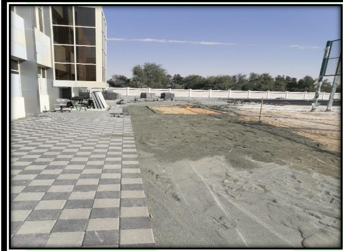
Interlocking Paving Tile Laying for School
