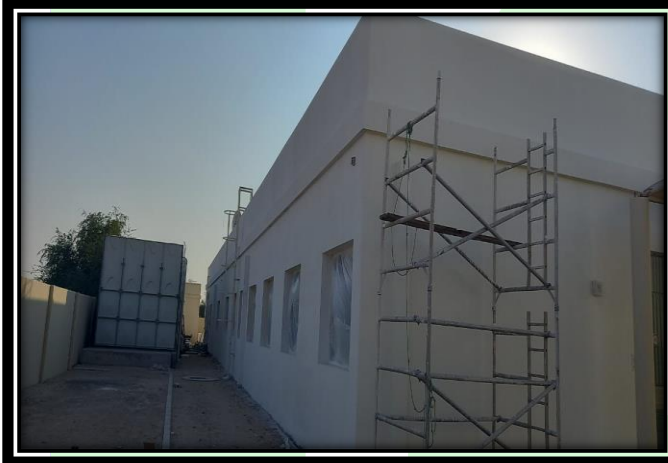
Internal and External Painting in School
