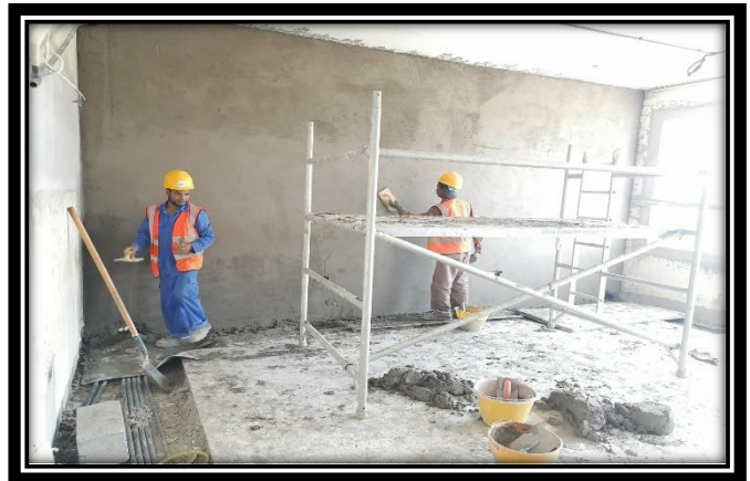
Block Work and Plastering in School
