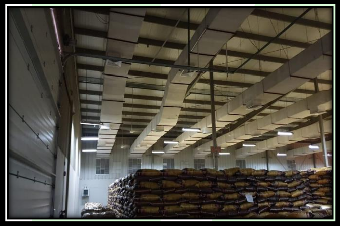
Sandwich Panel Replacement
