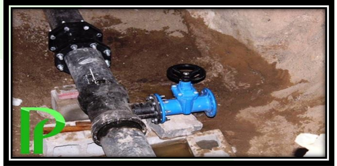
Bawadi Mall - D.I Main Line Modification Works
