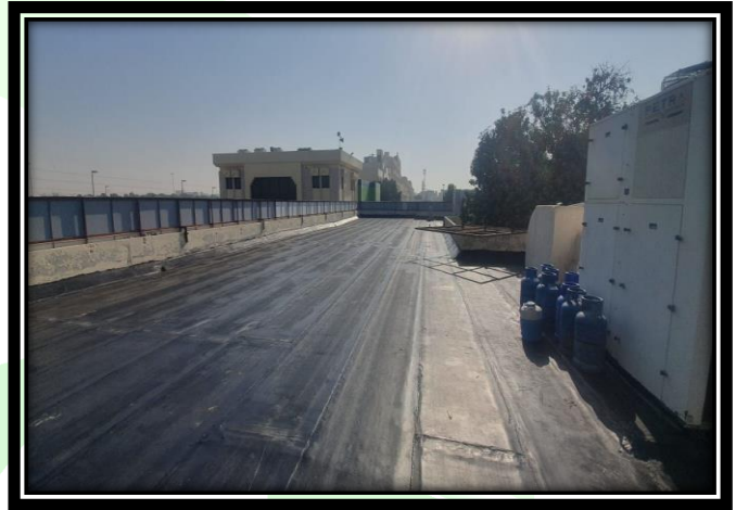
Roof Waterproofing
